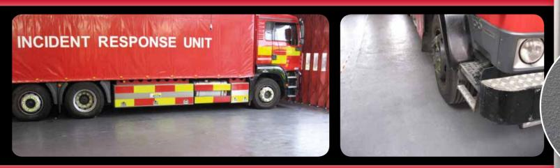
Richco Fire Brigade System has been specifically designed and manufactured for the installation onto appliance bay floors at fire stations. The finished system provides a hardwearing finish that tolerates the weight of the appliances whilst achieving the maximum anti-slip properties.
